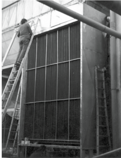
Duct Heater 4000 kW for Dehydration in the Agricultural Industry
