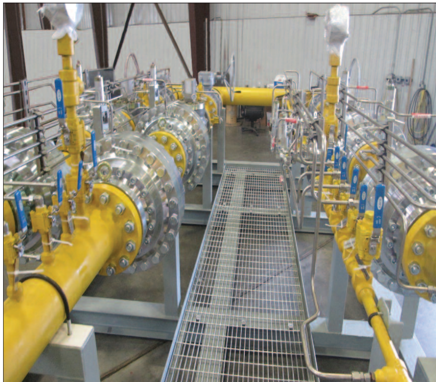
Wide-open monitor PCV arrangement
